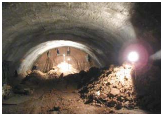
KALOTA - TUNEL CHENG WANGZHUANG
